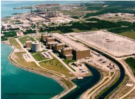
No 4 - Bruce 6,841 MW Canada
